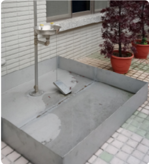
Liquid barrier installed in eye-washing equipment
