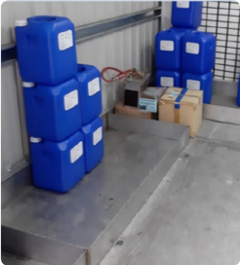
Liquid barrier installed in explosion-proof room
